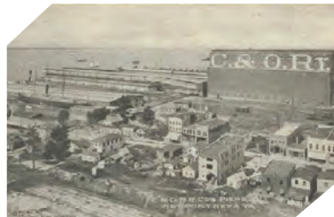
C&O Coal Piers at Newport News
